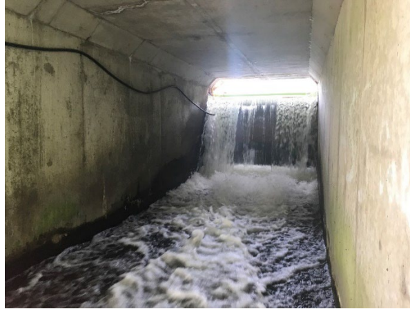
Photo 4: Middle Arden Dam: Looking Upstream at the Logs. Post Replacement. Water elevation is overtopping the top log.
