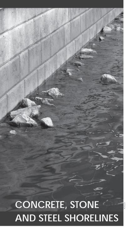
Structures made out of rock, concrete, metal and other materials were once commonly used when it was thought that the only way to combat erosion was to take a hard and aggressive approach. People began putting in retaining walls. These structures do work well in the short term to prevent erosion, but they ultimately do much more harm than good.
