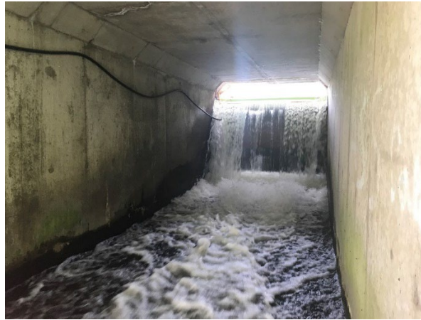
Photo 4: Middle Arden Dam: Looking Upstream at the Logs. Post Replacement. Water elevation is overtopping the top log.
